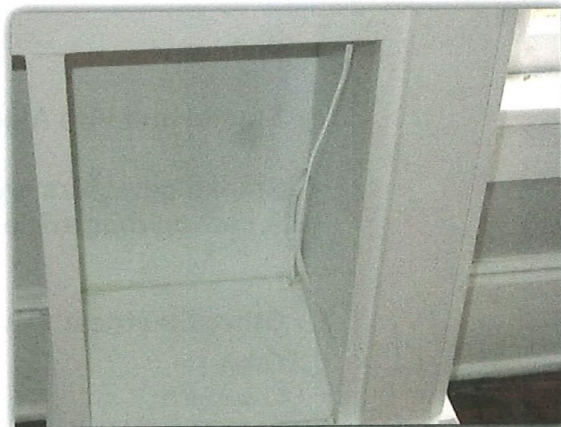
Wiring in NW Bedroom Not in Conduit
