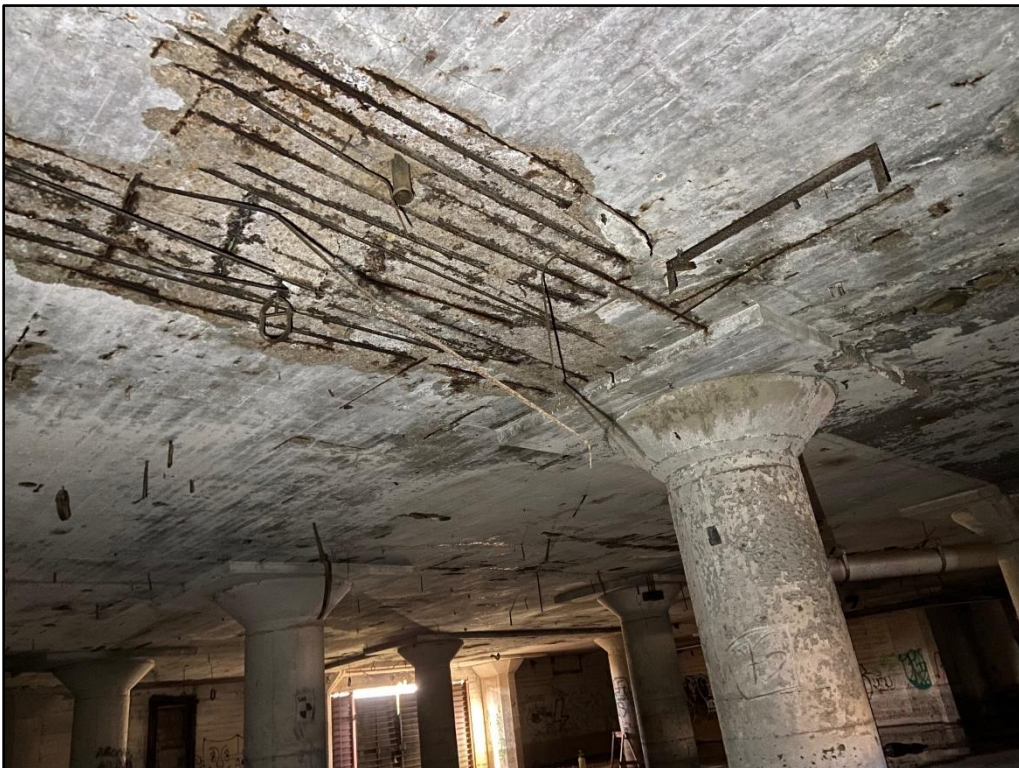
Photo 4: Spalled concrete with severely corroded rebar
