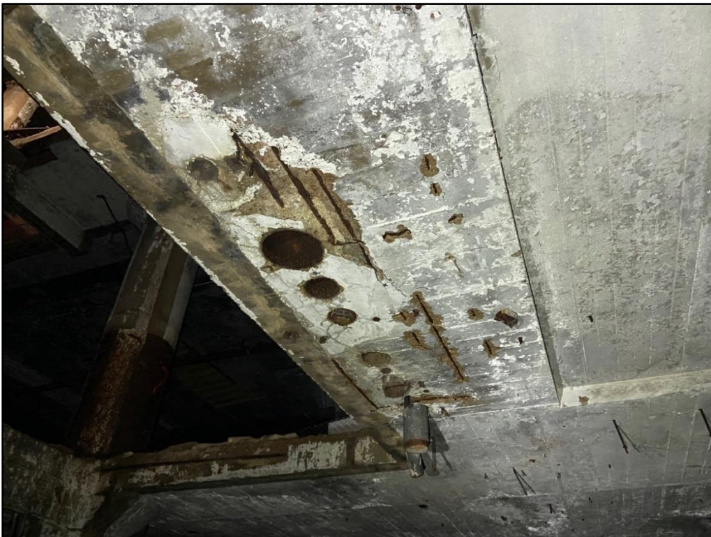
Photo 6: Various areas of spalled concrete in bottom and side of thickened slab at elevator core
