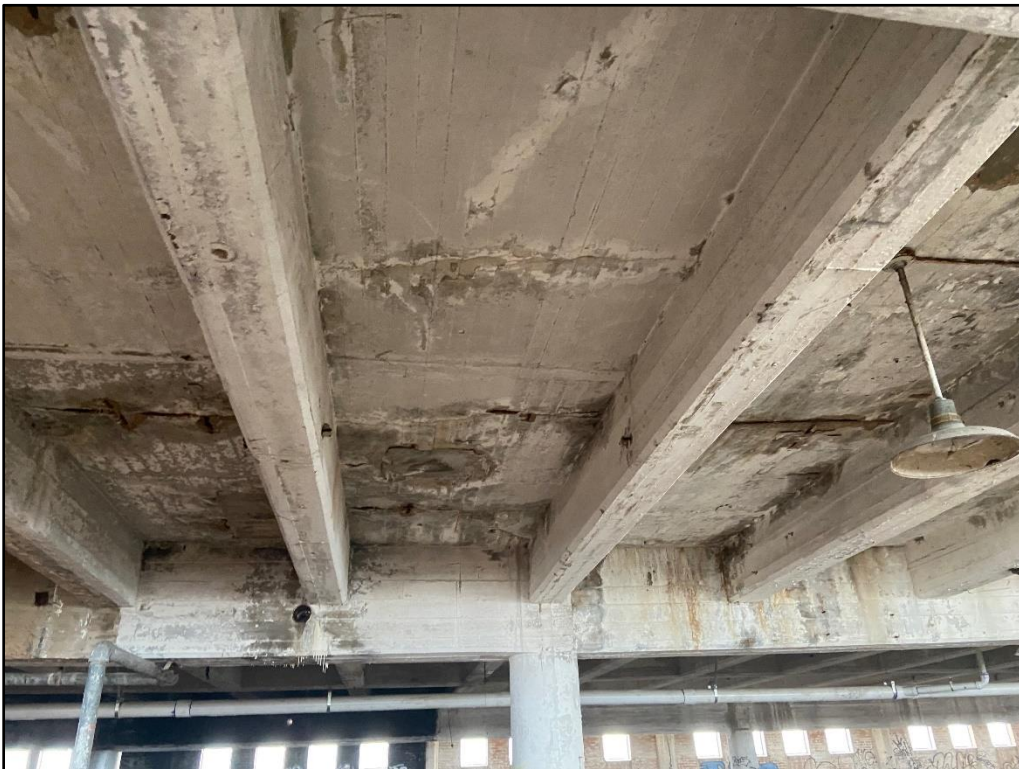
Photo 32: Various areas of spalled concrete and cracks in bottom of slab of varying size and length
