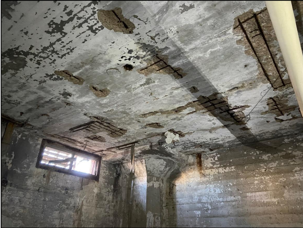
Photo 1: Various areas of spalled concrete in bottom of slab of varying size
