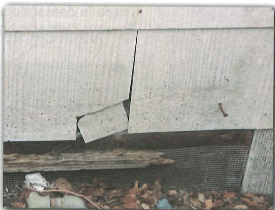
Damaged Siding at the South Side of House
