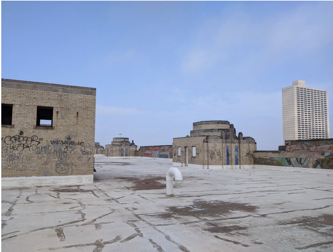
Fig. 12 – Photo of rooftop with failing temporary roof
