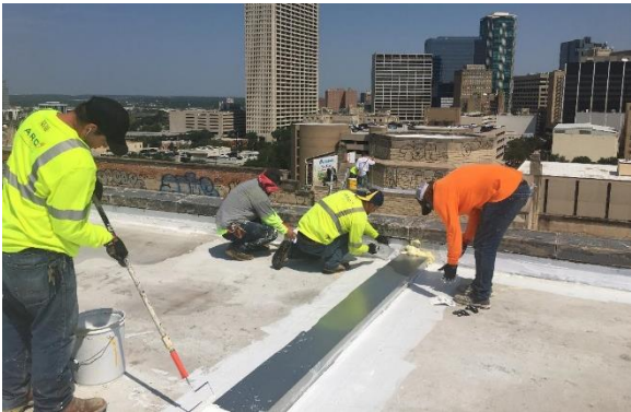
Figure 22 -- 8.20.18 -- Flashing & Expansion Joint Work on Penthouse
