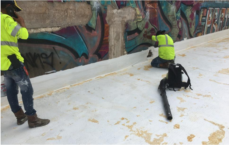
Figure 14 -- Touch-up Work on Emergency Drain Scuppers
