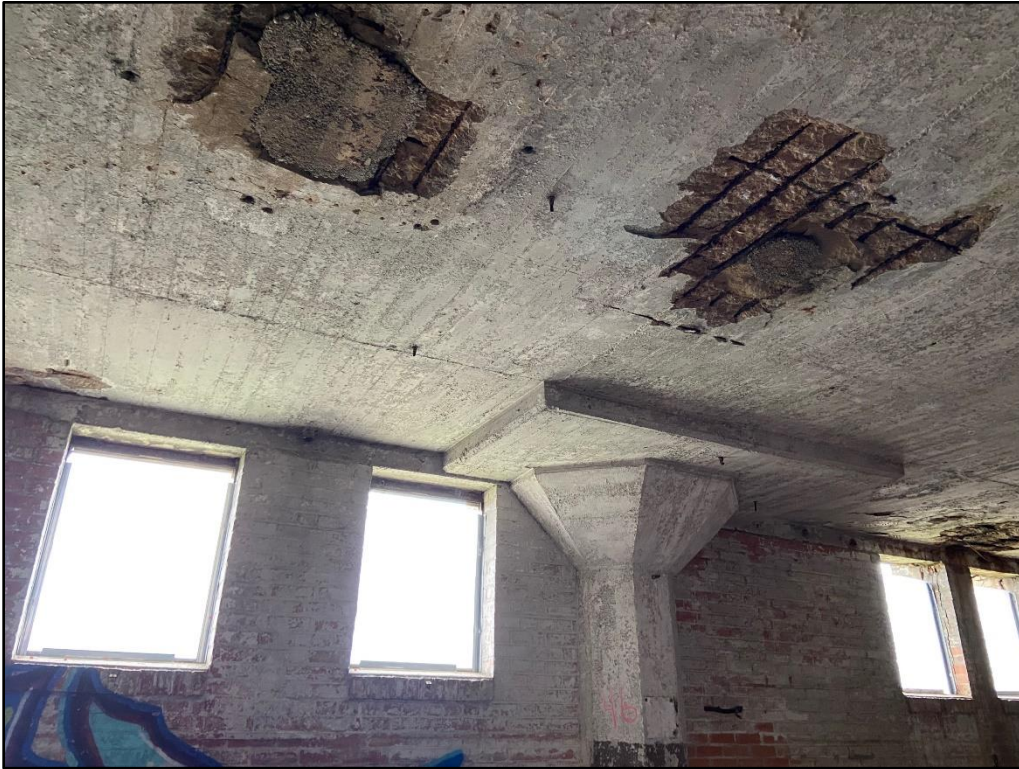
Photo 13: Example of deteriorated patchwork over areas of spalled concrete
