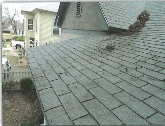
Hail Damaged Shingles
