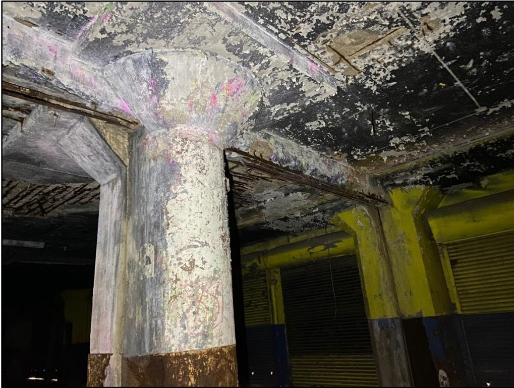
Photo 11: Spalled concrete with severely corroded rebar at bottom of beam
