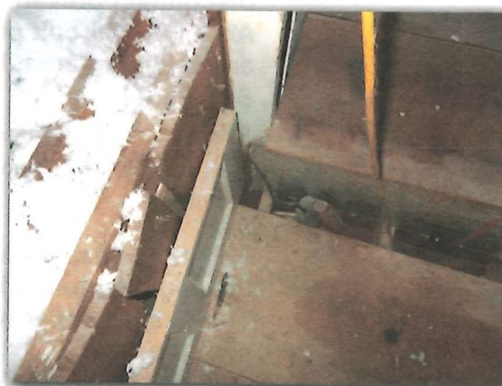
Wiring Connections Not in Junction Box Junction Box in Stairway Not Secured Ground/ARC Fault Circuit Interrupt Safety Protection
