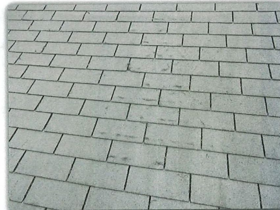
Hail Damaged Shingles
