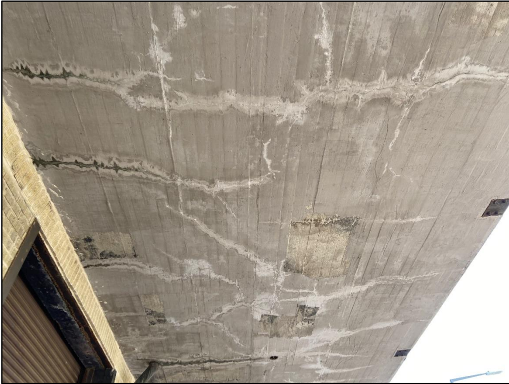
Photo 19: Various cracks in bottom of exterior north canopy of varying length
