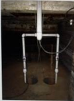
Installed Pumps & Drainage Piping West Basement Sump
