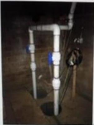
Installed Pumps & Drainage Piping East Basement Sump
