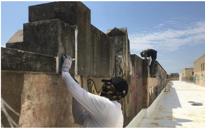
Figure 7 -- 9.6.18 -- South Parapet Limestone Cap Joint Sealant Prior to Mortar Dust Application
