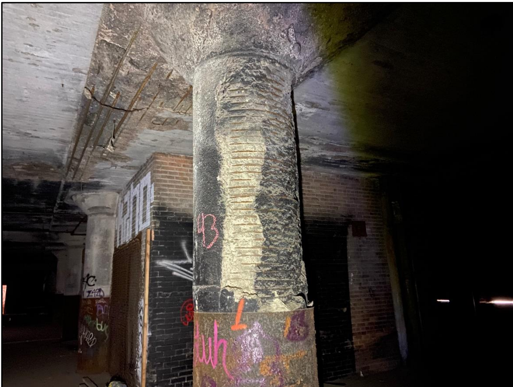
Photo 16: Spalled concrete at column, damaged column capital, and spalled concrete in bottom of slab
