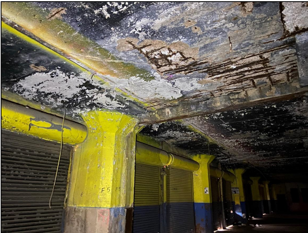
Photo 10: Spalled concrete with severely corroded rebar in bottom of slab
