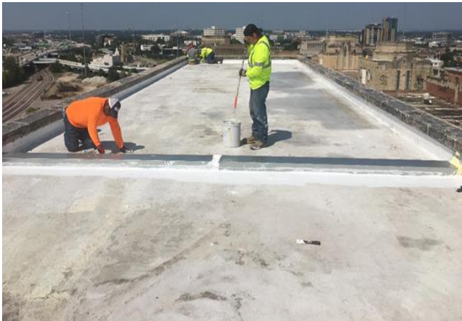
Figure 21 -- 8.20.18 -- Penthouse Expansion Joint Installation
