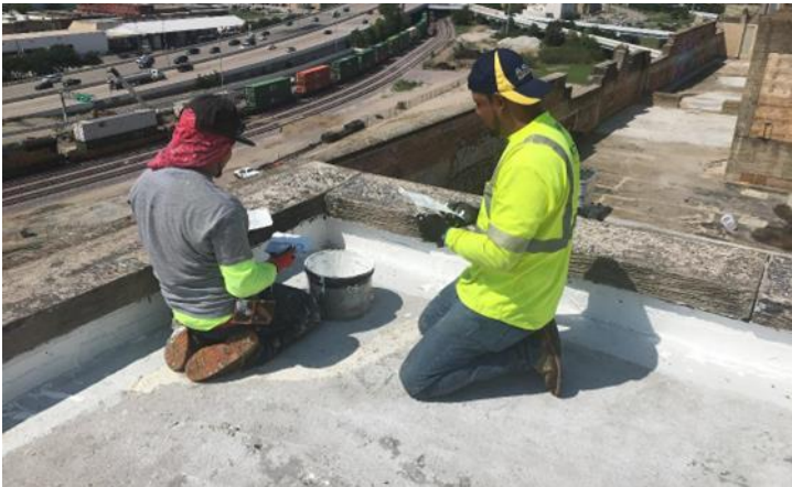
Figure 17 -- 8.20.18 -- Flashing of Parapet on a Penthouse
