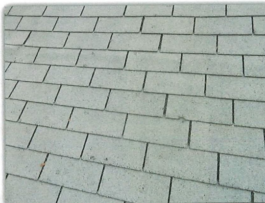
Hail Damaged Shingles
