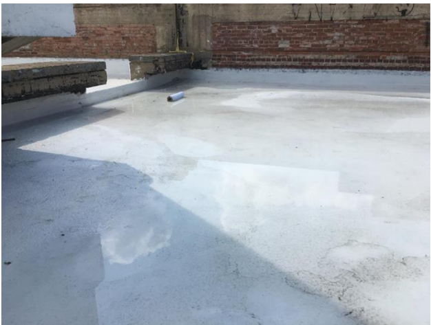
Figure 15 -- 9.7.18 -- Southeast Corner of Old Refrigerated Warehouse Area Showing Finished Flashing and Roof
