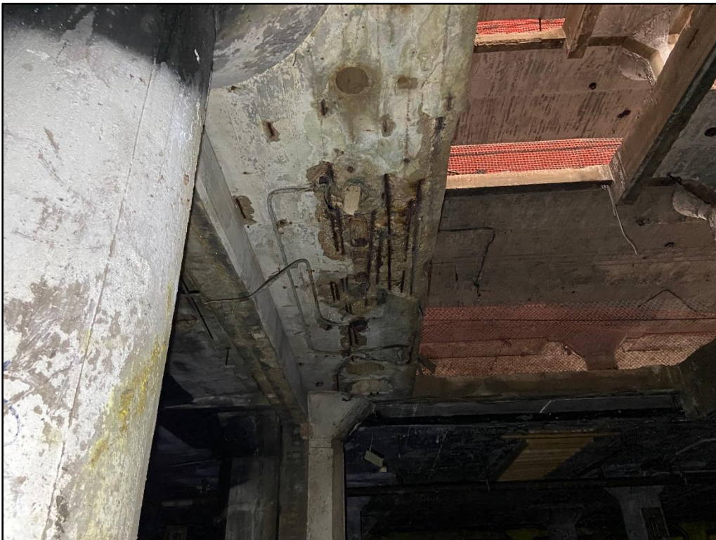
Photo 14: Severe deterioration in thickened slab around elevator core at existing floor openings
