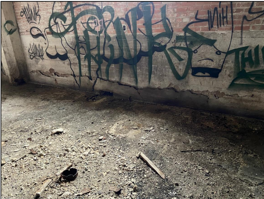
Photo 36: Concrete crack and spalled concrete at bottom of wall
