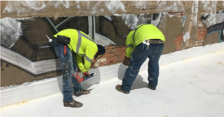
Figure 4 -- 9.5.18 -- Final Coat and Touch-up on Flashings at North Parapet Wall
