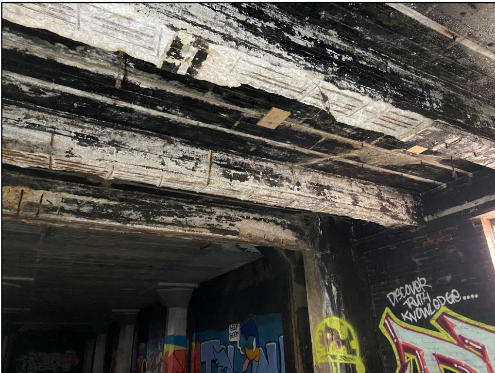
Photo 34: Spalled concrete and mildly corroded rebar in bottom and sides of roof beams
