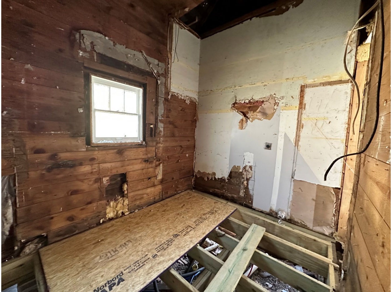
Figure 11 – Structural repairs to floor and foundation.
