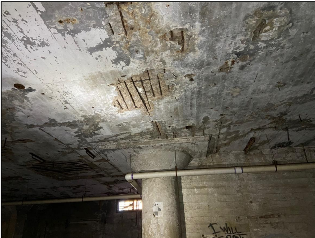
Photo 2: Various areas of spalled concrete in bottom of slab of varying size
