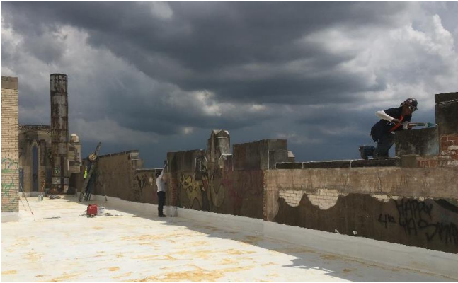
Figure 8 -- 9.6.18 -- Crew on Limestone Cap Joint Sealant Work
