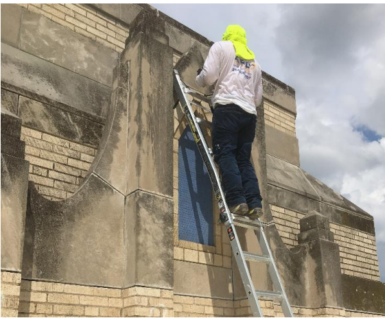
Figure 6 -- 9.6.18 -- Limestone Joint Sealant Work - NE Bungalow
