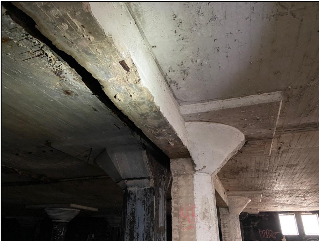
Photo 28: Spalled concrete with exposed, corroded rebar at bottom of beam
