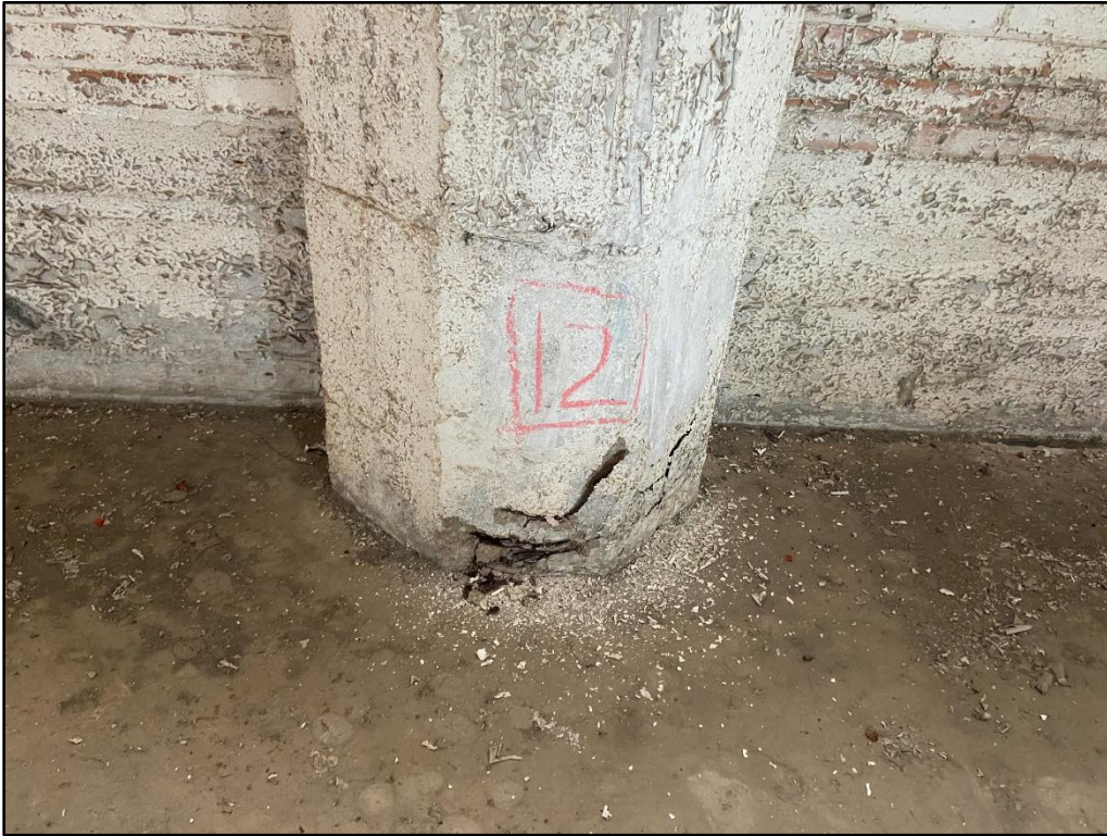
Photo 23: Spalled concrete with exposed, corroded rebar at bottom of column
