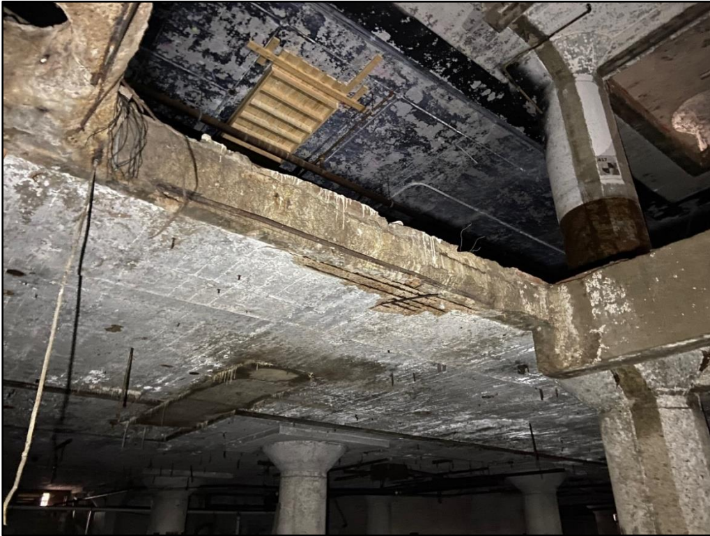
Photo 5: Various areas of spalled concrete in bottom and side of thickened slab at elevator core
