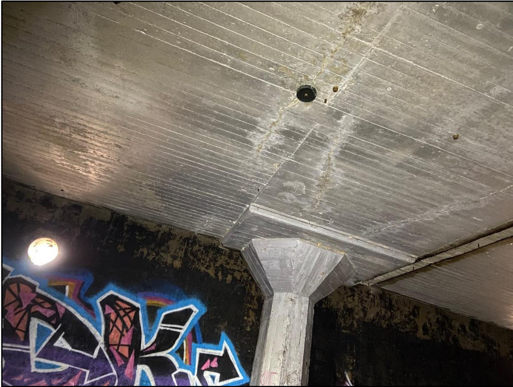
Photo 33: Various cracks in bottom of slab of varying length
