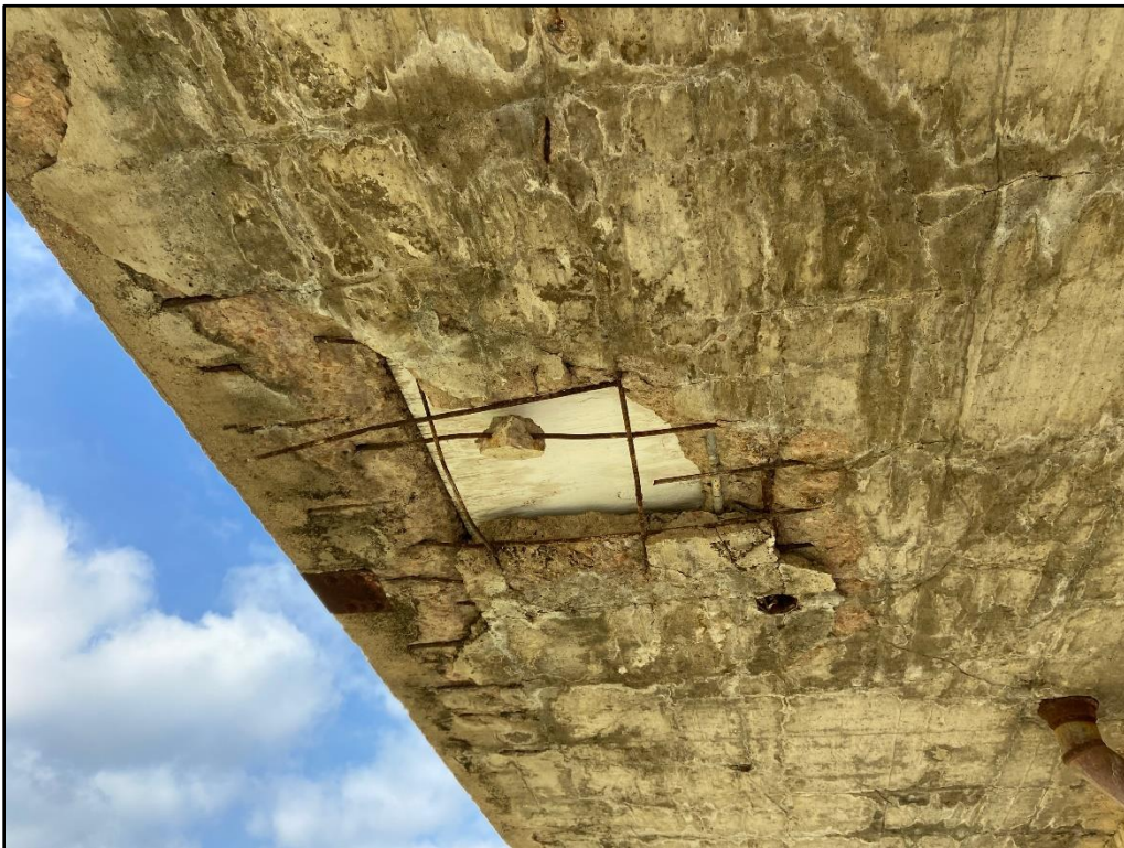
Photo 18: Missing concrete and exposed rebar in exterior south canopy
