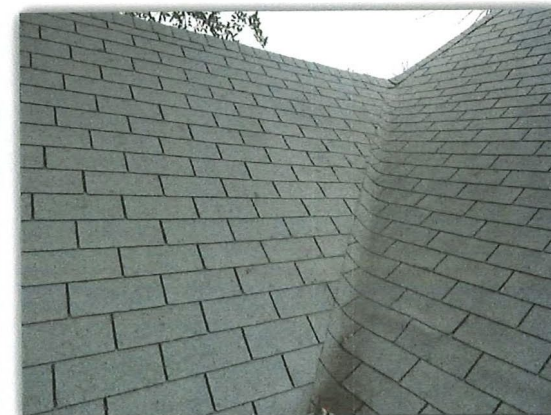
Hail Damaged Shingles
