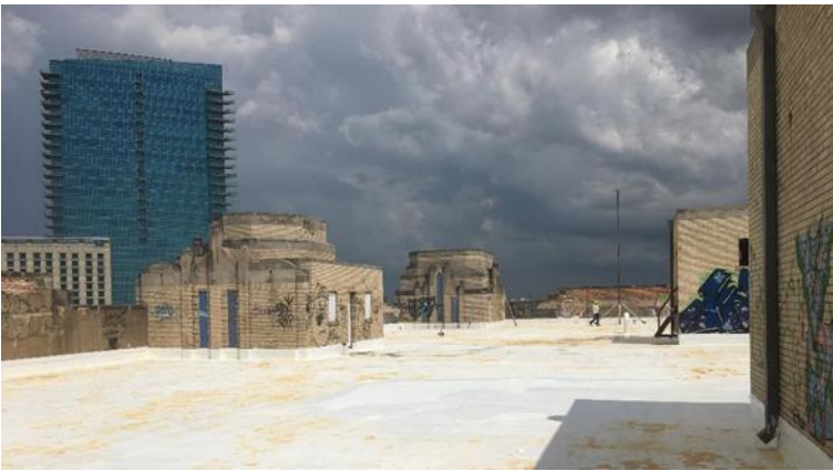
Figure 9 -- 9.6.18 -- North Side of Roof Looking East – Shows Completed Flashing and Final Top “White” Coat of Roofing
