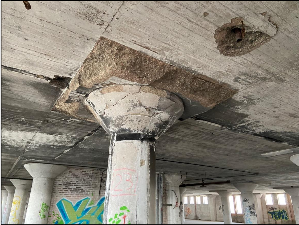
Photo 25: Spalled concrete in column capital and drop panel
