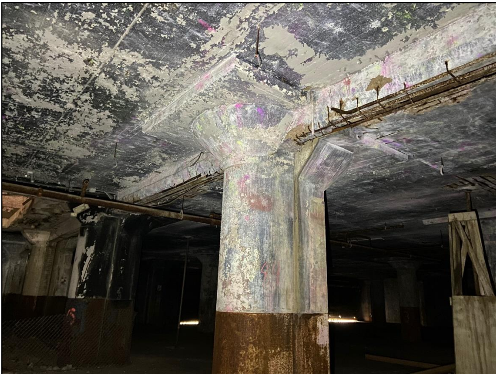
Photo 12: Spalled concrete with severely corroded rebar at bottom of beam
