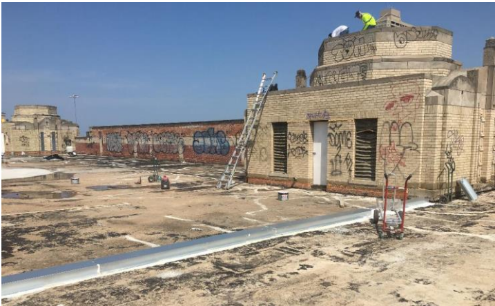
Figure 18 -- 8.20.18 -- Expansion Joint Cover Installed - Flashing Work on Bungalow
