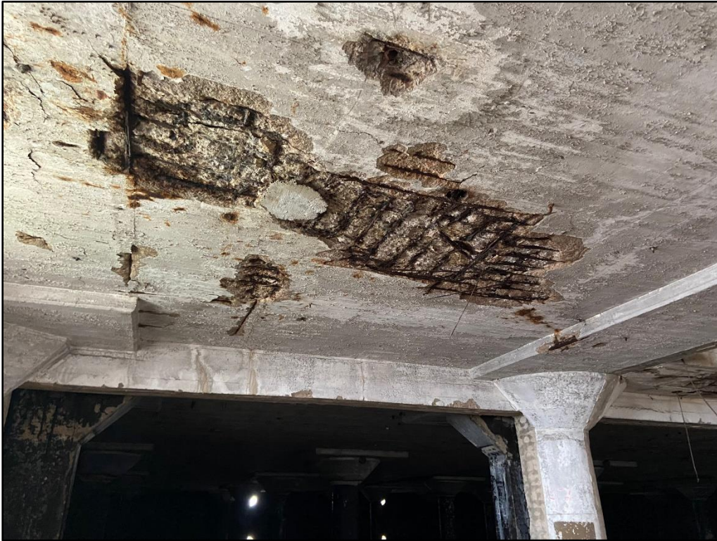
Photo 29: Spalled concrete with severely corroded rebar
