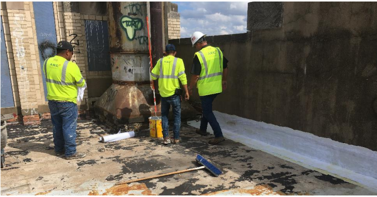
Figure 2 -- 9.4.18 -- Determining How to Install Flashing Around the Main Flue Stack for Coating
