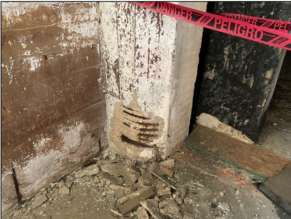
Photo 26: Spalled concrete with exposed, corroded rebar at bottom of column
