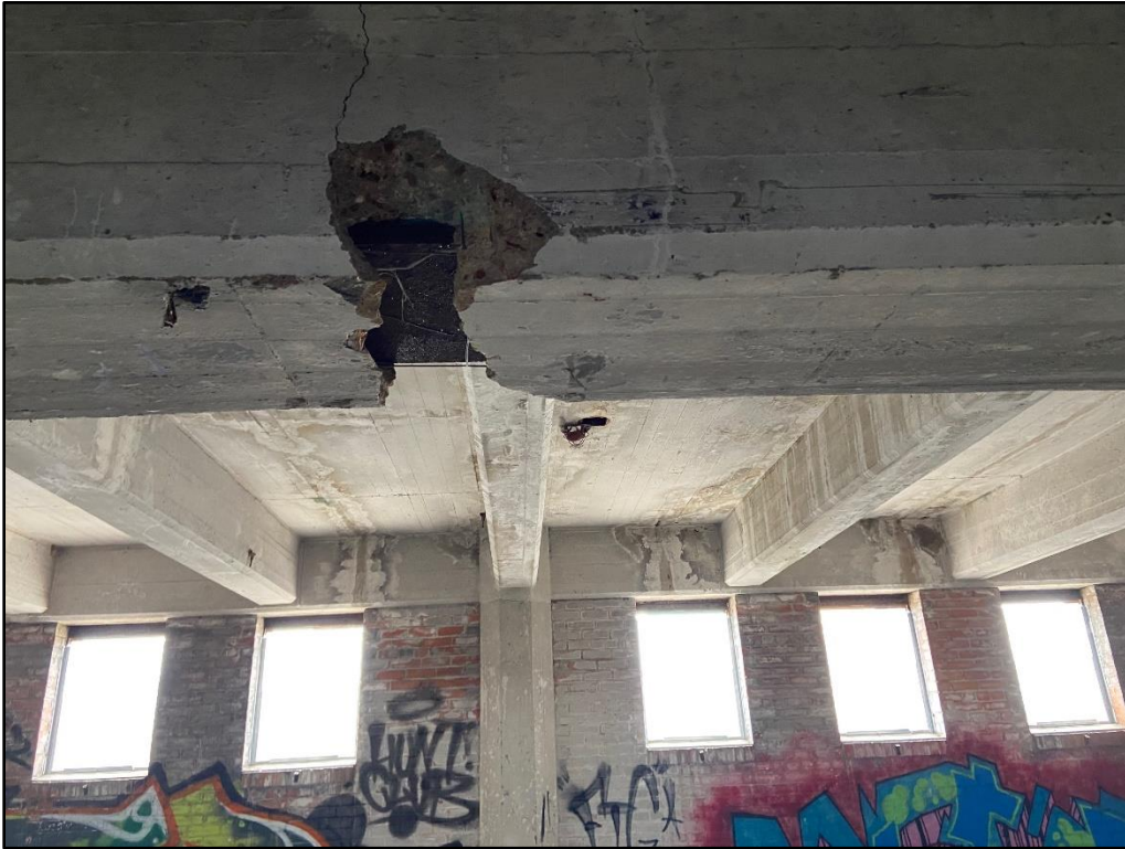
Photo 37: Spalled concrete and exposed wide flange girder
