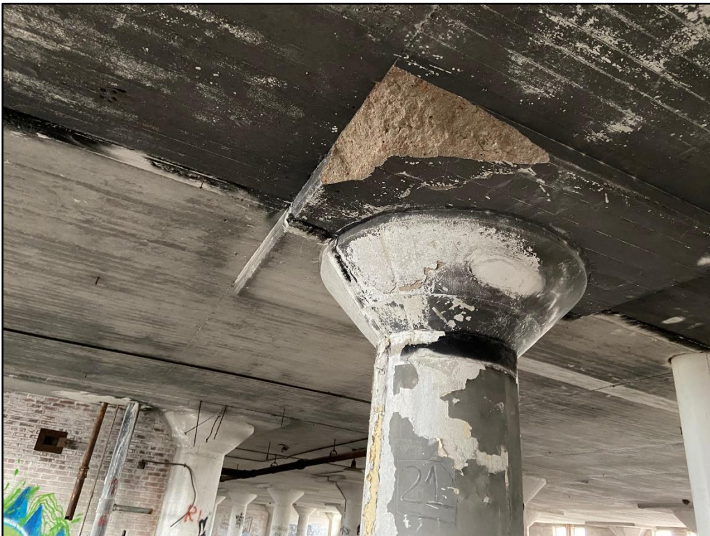
Photo 24: Spalled concrete in column capital and drop panel
