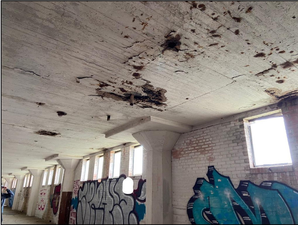
Photo 27: Various areas of spalled concrete in bottom of slab of varying size
