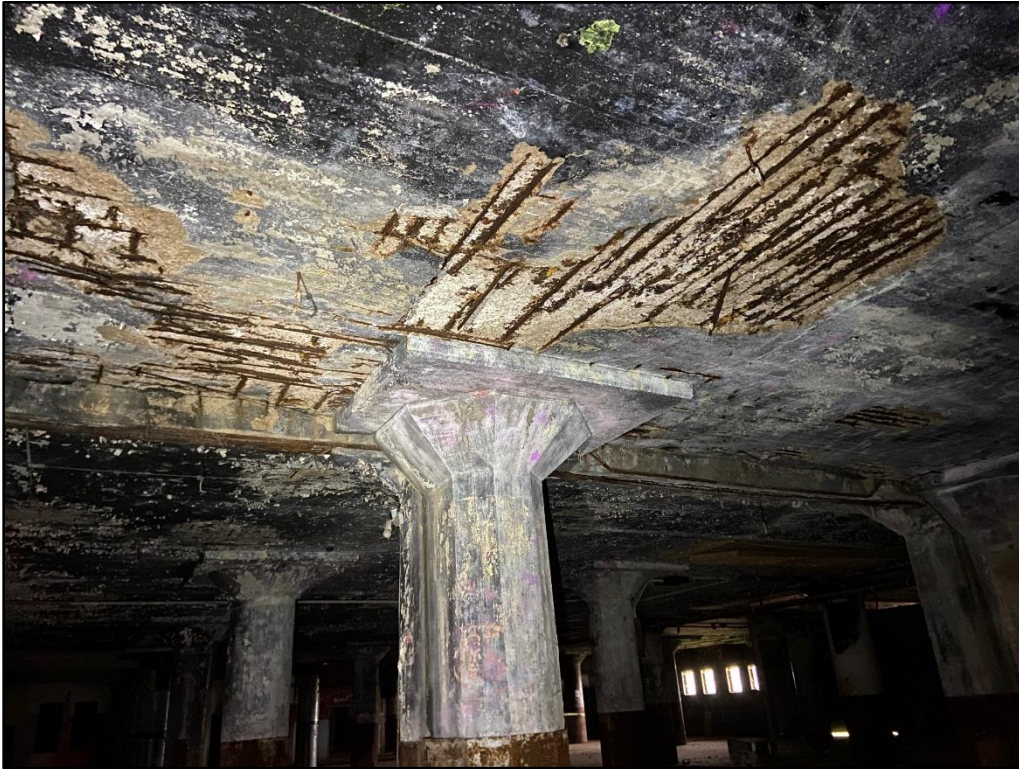
Photo 9: Spalled concrete with severely corroded rebar in bottom of slab
