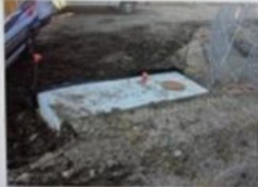
New Storm Sewer Inlet by City
