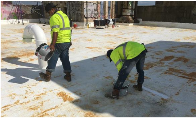
Figure 13 -- 9.7.19 -- Touch-up Work - Treating any Deck Cracks Which May Have Been Missed Earlier
