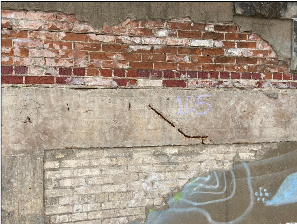
Photo 38: Spalled concrete and exposed rebar on inside face of parapet
