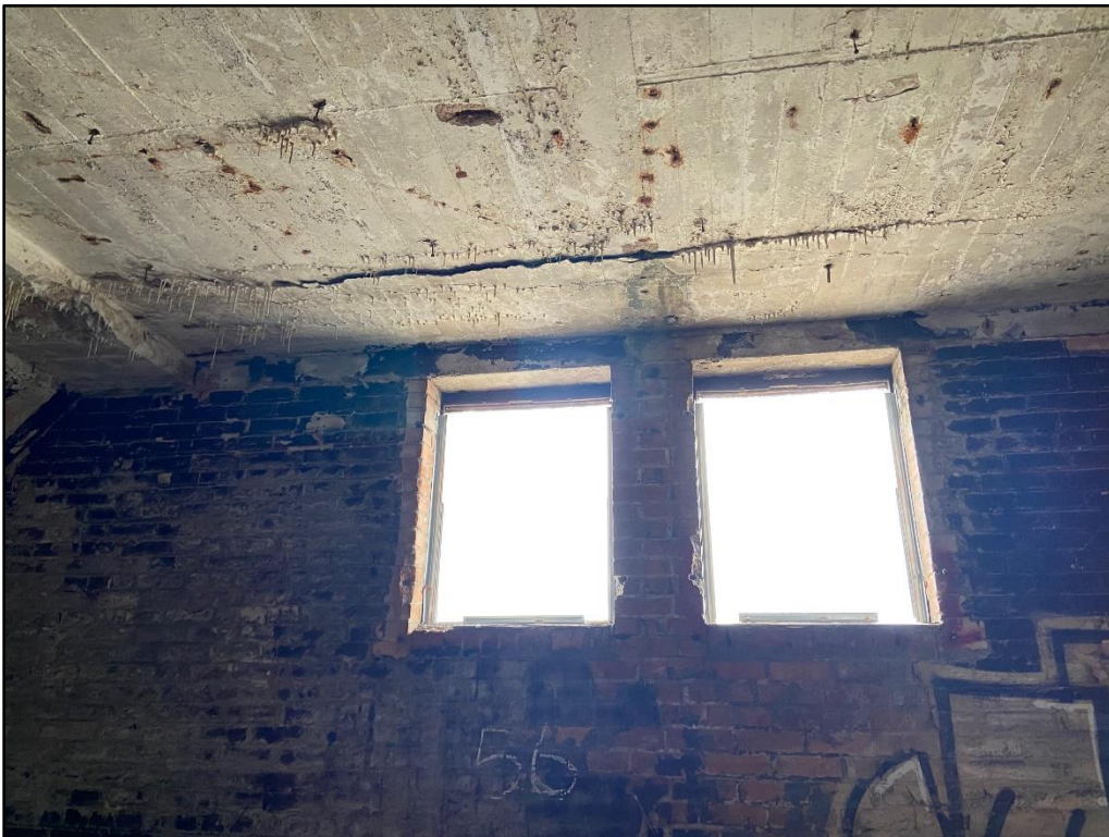
Photo 30: Crack in bottom of floor slab
