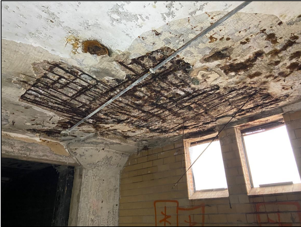
Photo 21: Spalled concrete with severely corroded rebar
