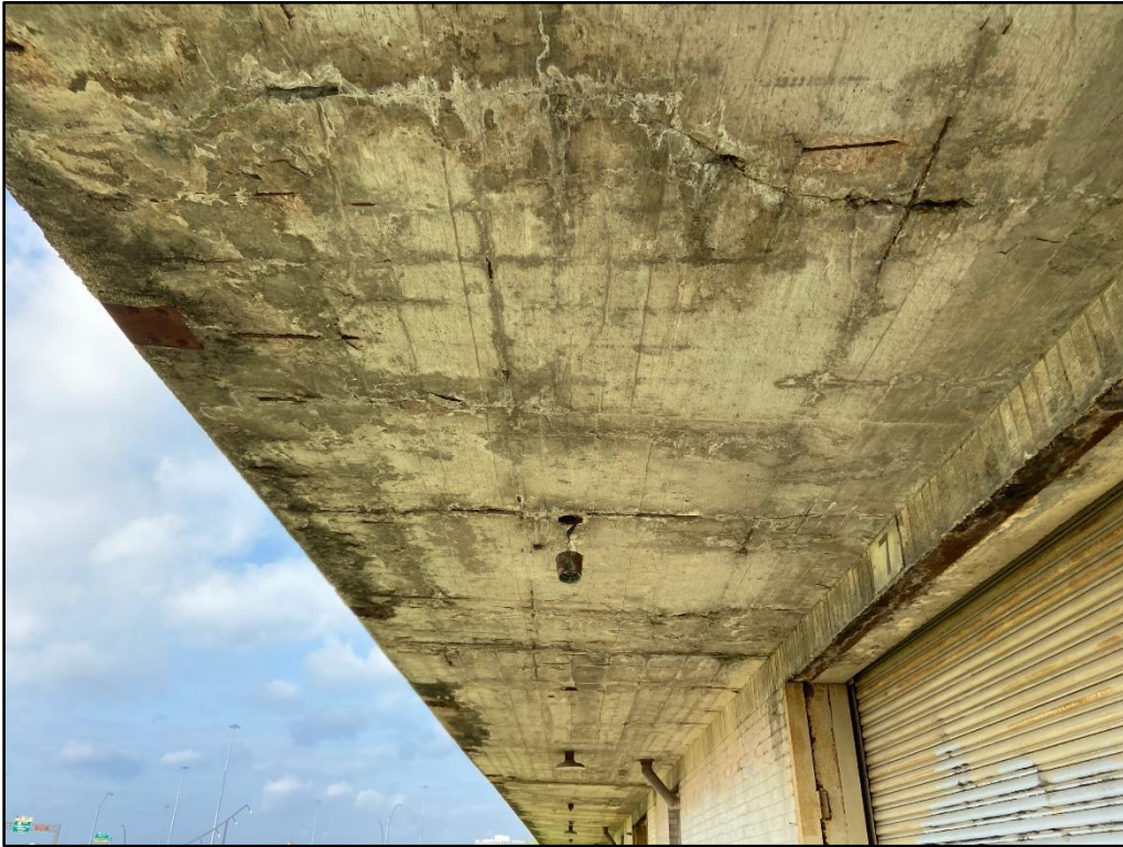
Photo 17: Various areas of spalled concrete and cracks in bottom of exterior south canopy of varying size and length
