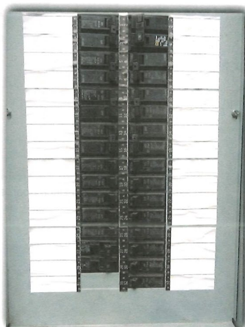
Service Panel Breakers Not Labeled
