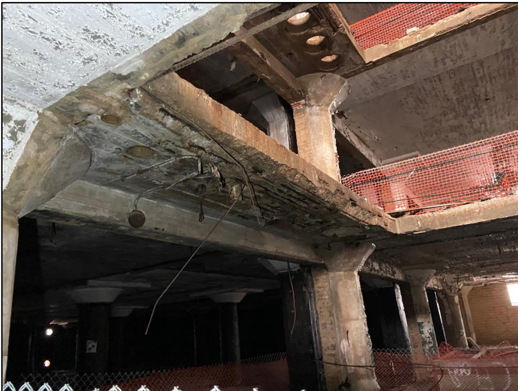
Photo 22: Severe deterioration in thickened slab around elevator core at existing floor openings
