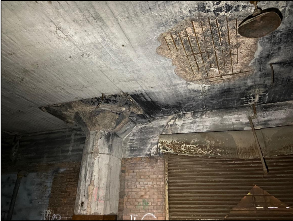
Photo 15: Spalled concrete in bottom of floor slab, damaged column capital and drop panel
