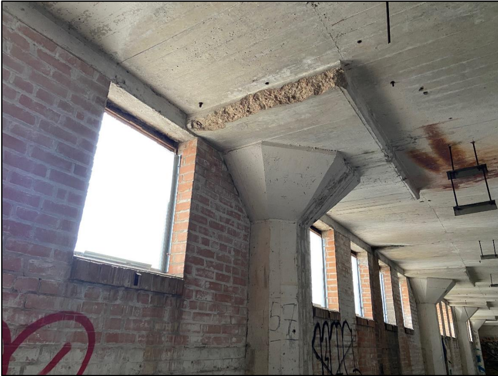
Photo 31: Spalled concrete in column capital and drop panel
