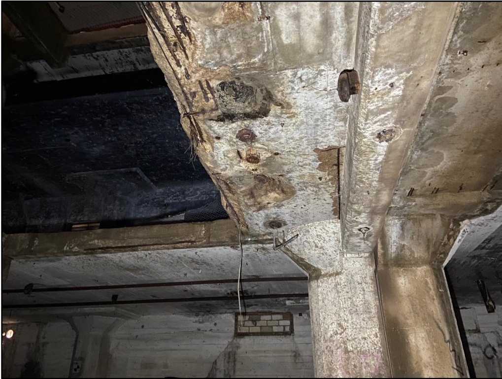
Photo 7: Severe deterioration in thickened slab around elevator core at existing floor openings
