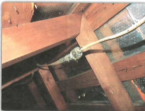
Wiring Connections Not in Junction Box Junction Box in Stairway Not Secured Ground/ARC Fault Circuit Interrupt Safety Protection
