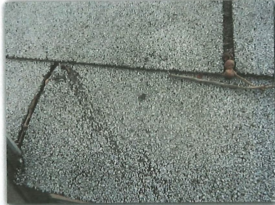
Damaged Shingles
