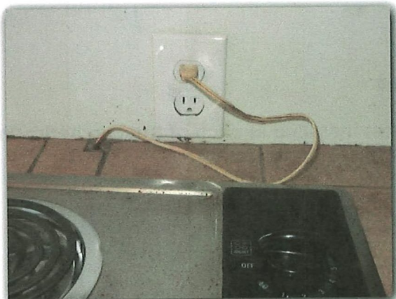
Improper Kitchen Wiring
