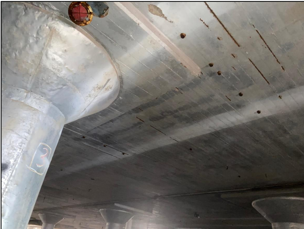
Photo 20: Example of exposed, corroded rebar with no apparent cover in bottom of floor slab
