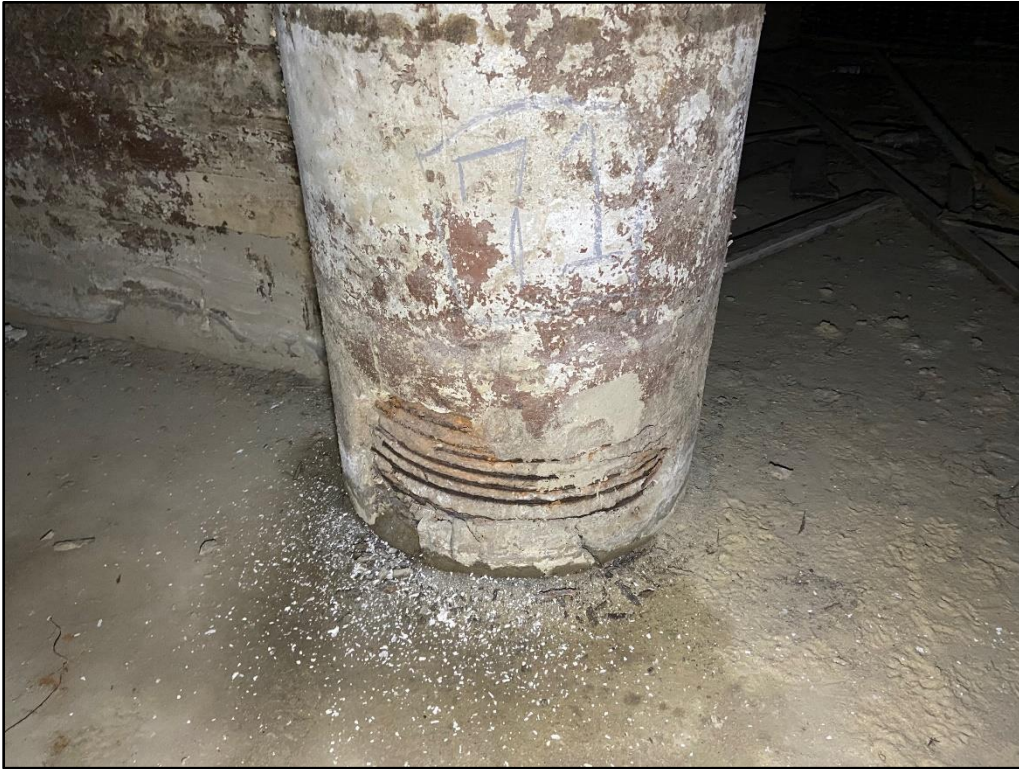
Photo 3: Spalled concrete and exposed, corroded rebar at bottom of column
