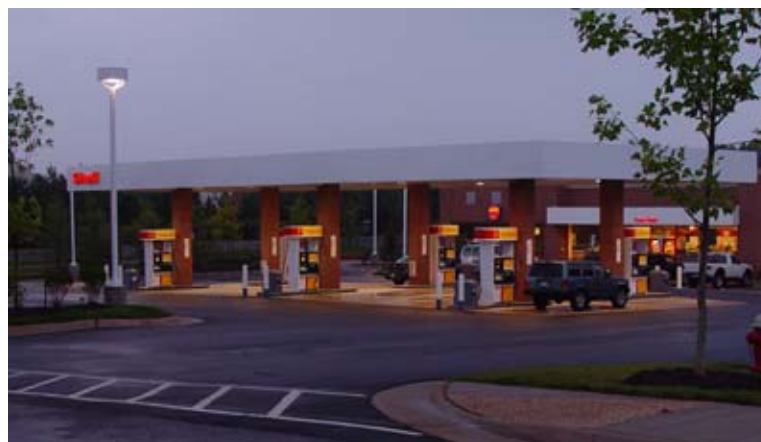
Example of service station down lighting
