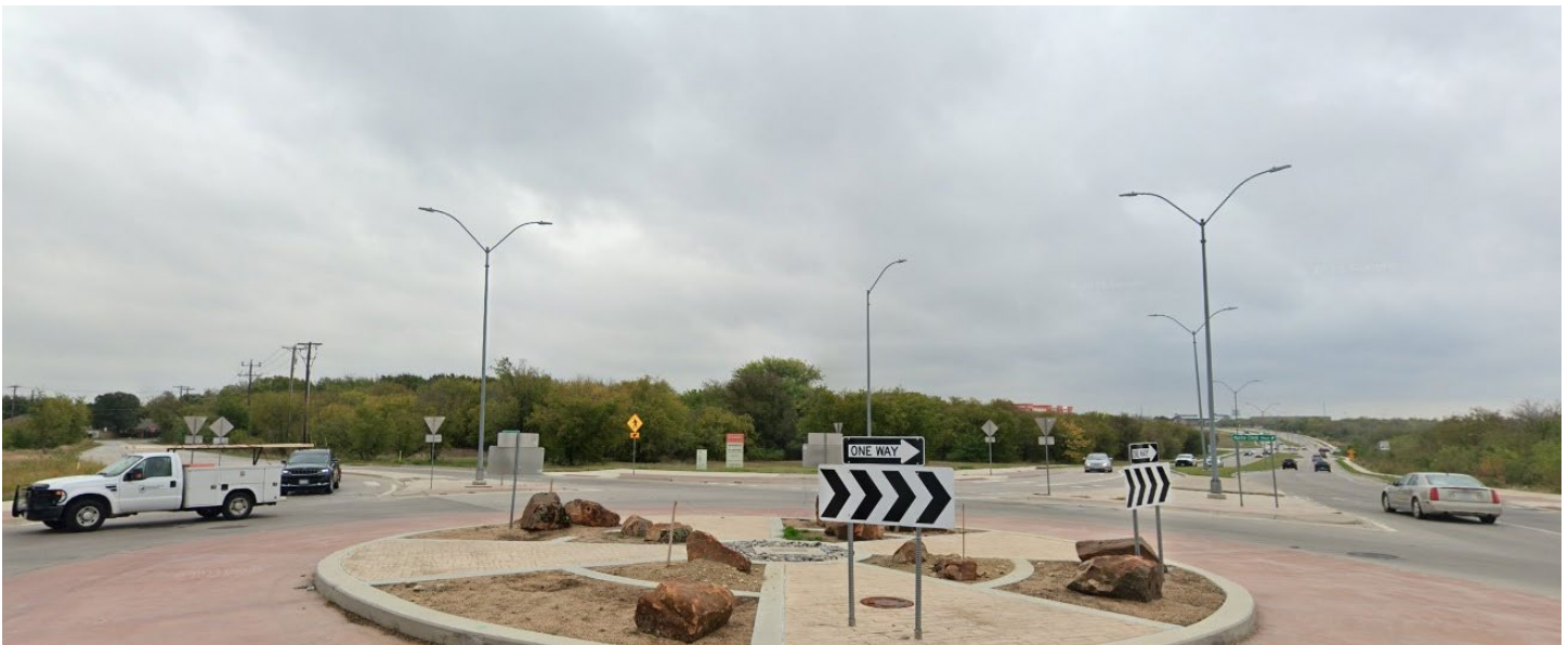
Northwest corner (Marine Creek Parkway & Cromwell Marine Creek Road roundabout)
