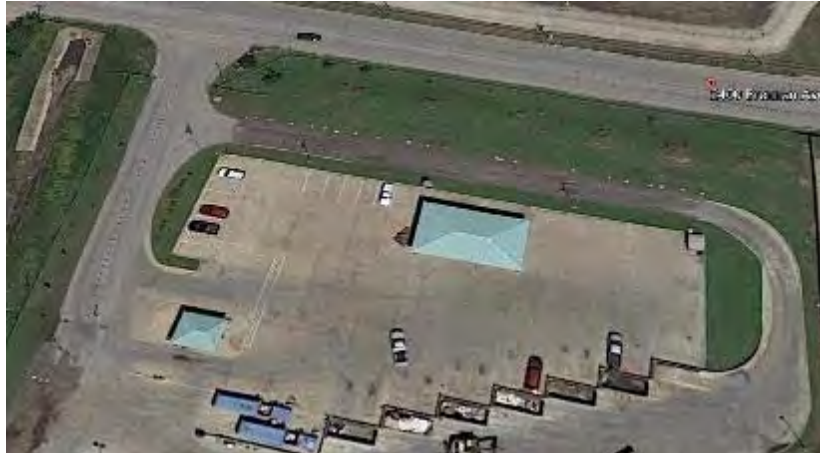
Figure 4-9 Brennan Drop-off Station
