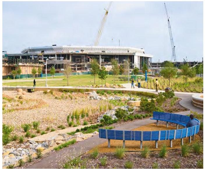
Figure 4-18. The Green at College Park on the University of Texas at Arlington campus boasts green infrastructure that captures 25 percent of stormwater and reduces sediment by 80 percent, photo from University of Texas at Arlington.
