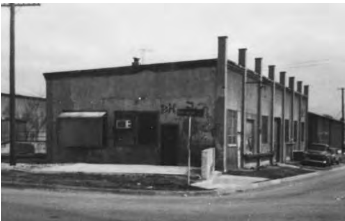
Figure 2-9. A building in Niles City (incorporated into the City of Fort Worth in 1911) shows how historical land use change can hide potential contamination on a property. This building was once a horse collar factory, Patterson’s Garage, a monument company, a broom company, then a storefront, photos from the University of North Texas Libraries, Portal to Texas History.
