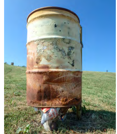
Figure 6-11. When the city took ownership of Echo Lake Park, some of the trash bins were in bad shape. Using the inventory, the city can set a replacement schedule for bins to ensure this does not happen in the future, photo by City of Fort Worth.
