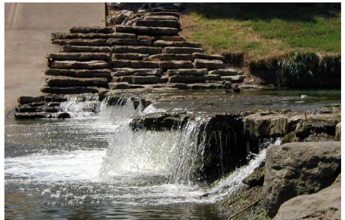
Figure 4-4. Water flowing on the Trinity River, photo by City of Fort Worth.
