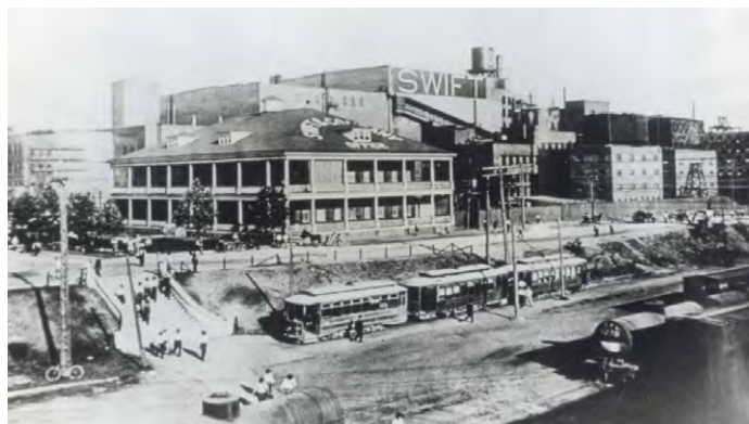
Figure 2-24. Historical industrial operations have led to present-day site contamination that the City of Fort Worth is addressing.
