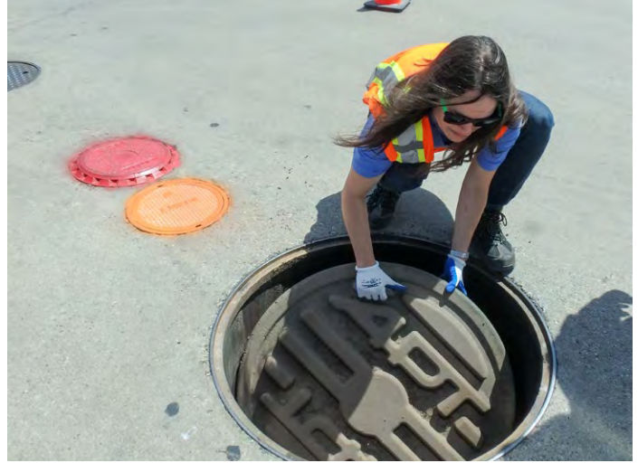
Figure 3-5. An Air Quality Section staff member inspects an underground storage tank at a gas station, photo by City of Fort Worth.
