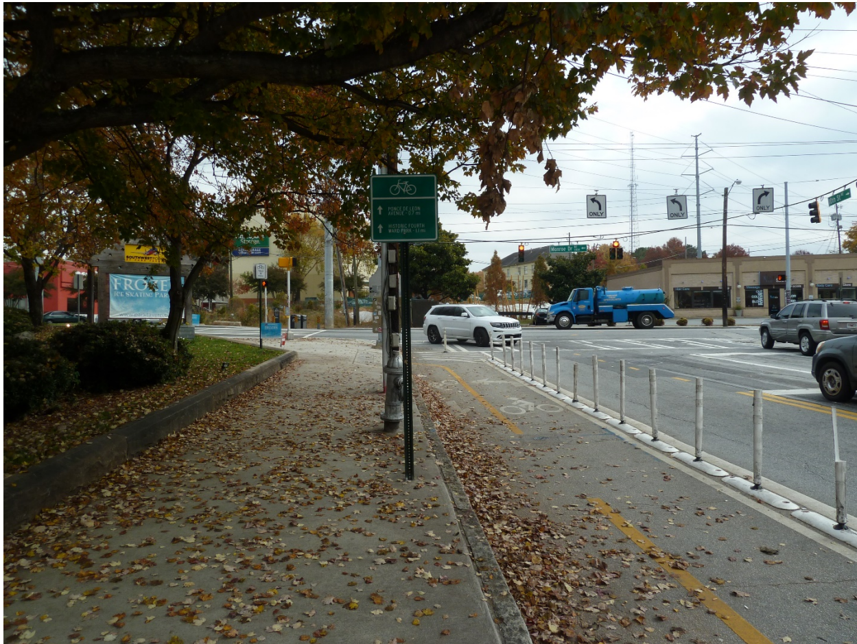
Figure 4-34. A Separated Bicycle Lane with Leaf Debris
