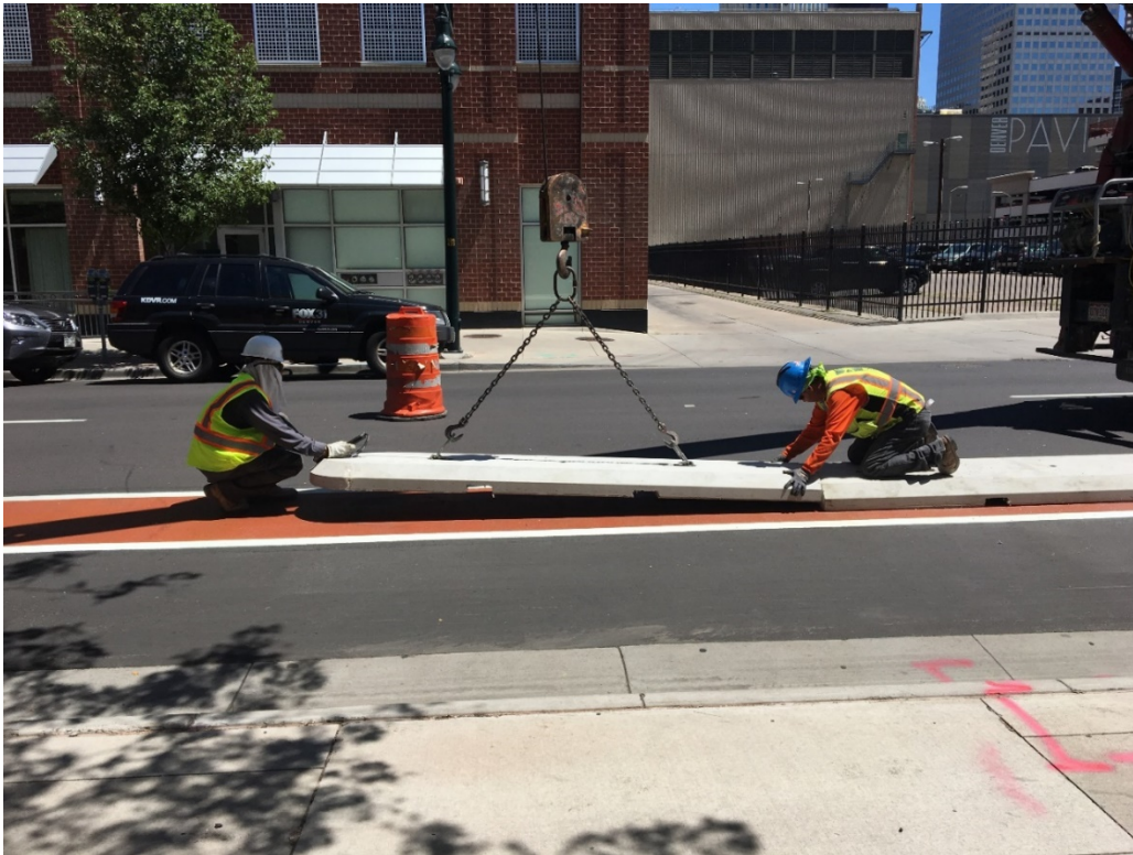
Figure 4-33. Installation of a Separated Bicycle Facility
