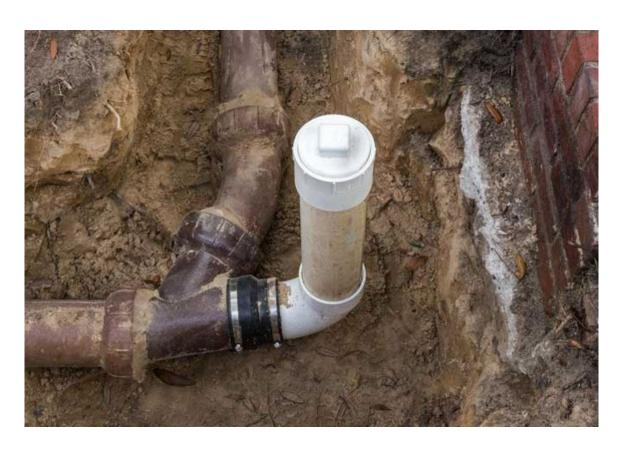
Sanitary sewer service will not be interrupted. New sewer cleanouts will be installed at the property line.
