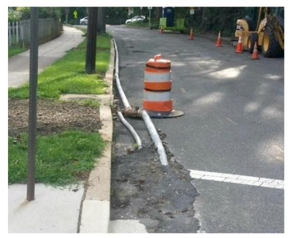
The temporary water line ensures that you are not without water during construction. In the summer months the continuous flow keeps the water from becoming stagnant in the aboveground line.
