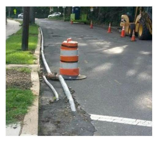
The temporary water line insures that you are not without water during construction. In the summer months the continuous flow keeps the water from becoming stagnant in the above-ground line.
