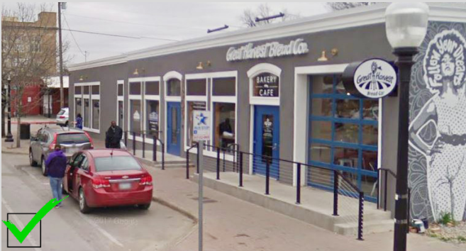
Use windows as character defining feature.
