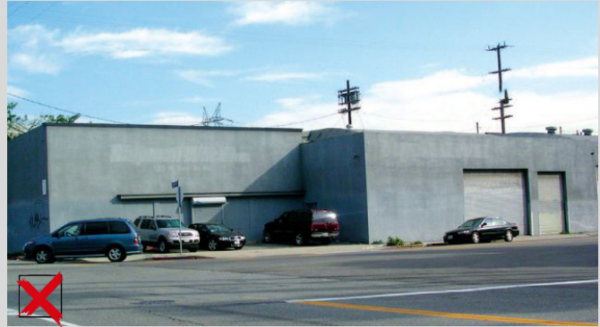
Lack of windows, architectural detail, or facade treatment creates dull and monotonous façade.
