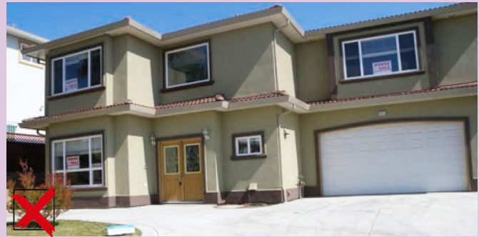
Excessive paving in this front yard creates a barren, undesirable street.
