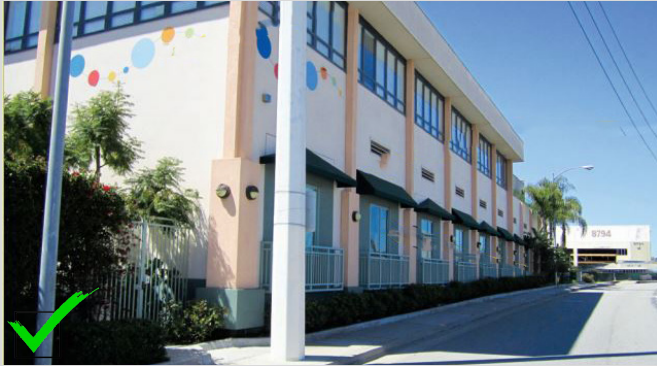
Colors, well-designed trim and detail, and ground floor windows facing the street provide visual interest.
