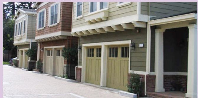
Locate the garage door behind the dwelling unit, preferably accessed from an alley or internal driveway.
