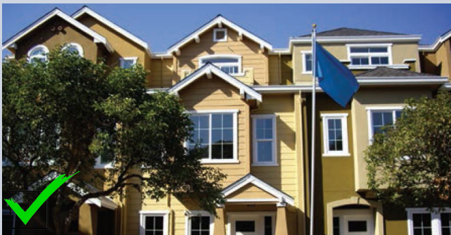
Upper stories articulated to break up the facade and minimize the appearance of mass.
