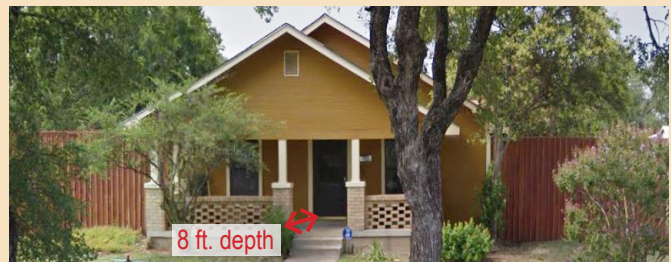
Consistent with the architecture of the house and a minimum 8 feet in depth.
