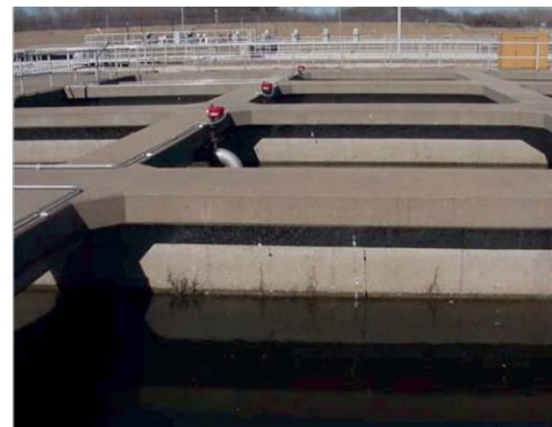
Traveling and Deep Sand Bed Filters
