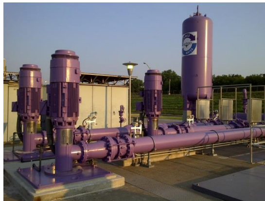
Village Creek Reclaimed Water Pump Station
