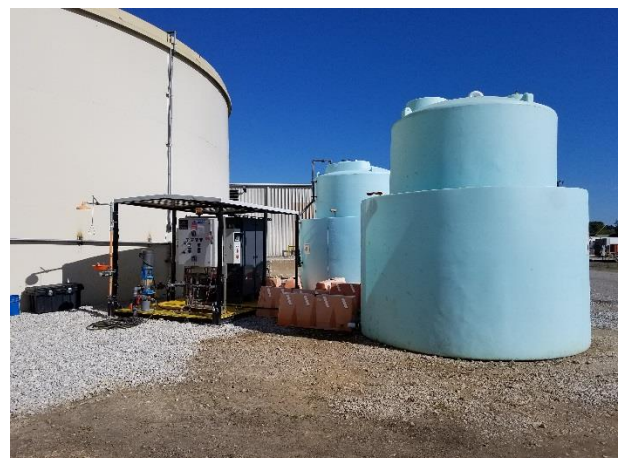
Chlorine Dioxide Treatment System
