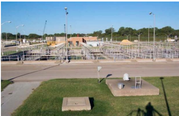
Traveling and Deep Sand Bed Filters
