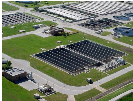
Chlorine Contact Basin
