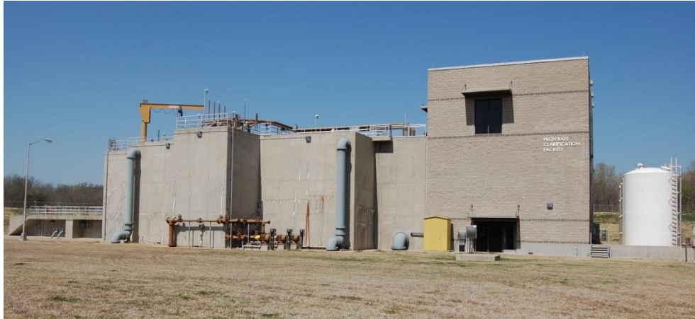
High Rate Clarifier Building
