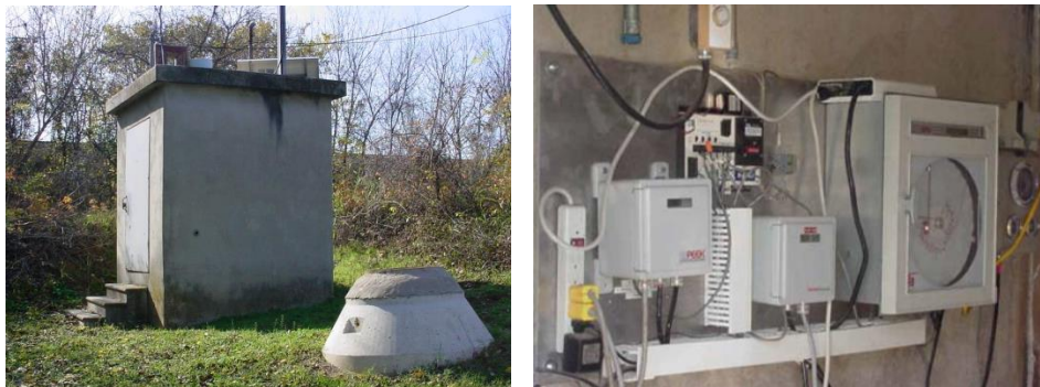
Metering Station and Equipment
