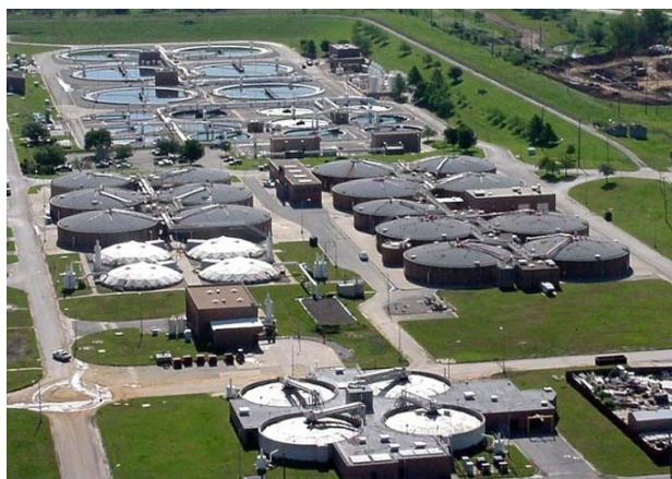
Anaerobic Digesters and DAFTs
