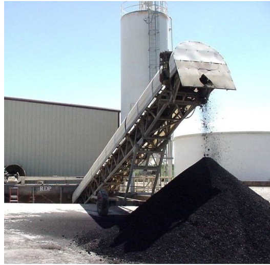
Lime Storage Silo & Pug Mill
