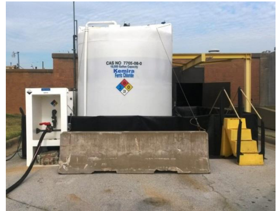
Ferric Chloride Station
