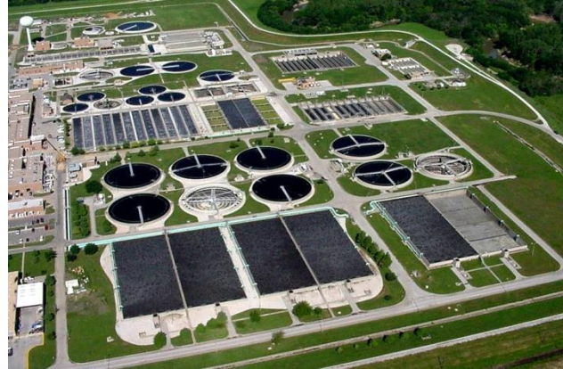
Aeration Basins and Final Clarifiers
