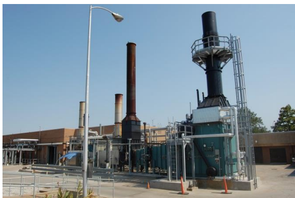
Heat Recovery Steam Generator & Duct Burner
