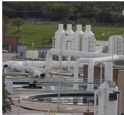
Covered Thickeners, Air Scrubbers, and Biofilters
