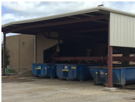
Grit Removal Facility
