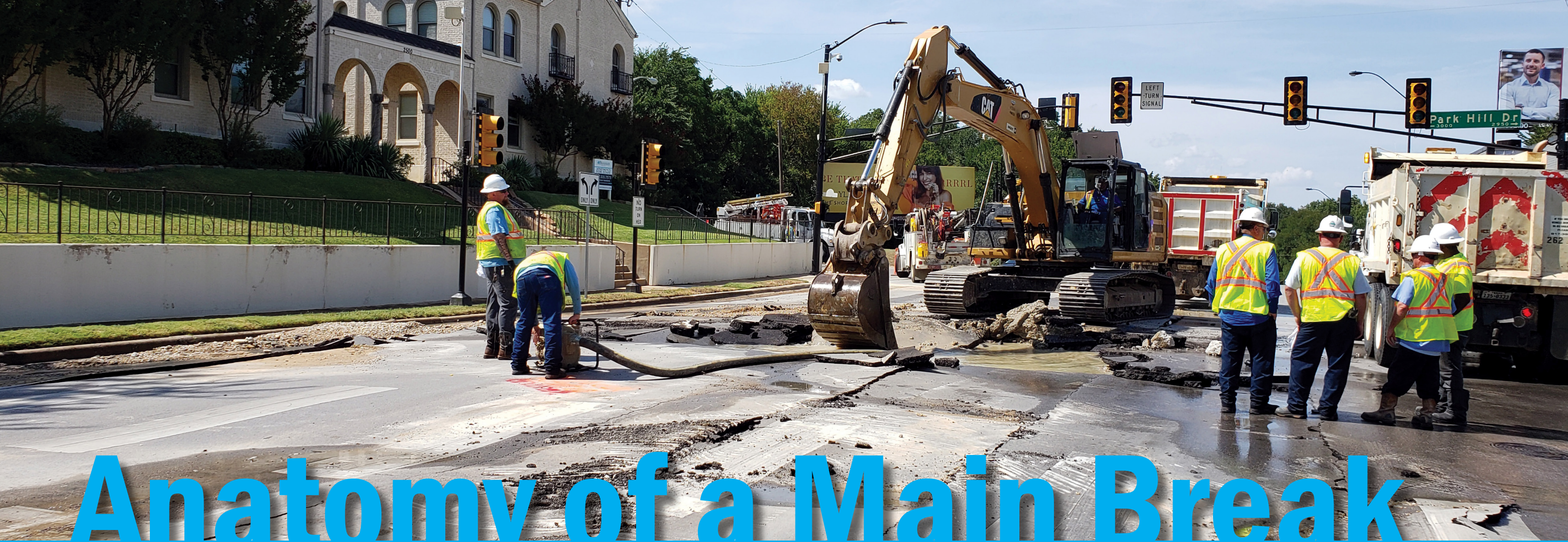
📷 Field Operations employees pump water out from the hole where a 63-year-old 24-inch cast iron water main broke.
